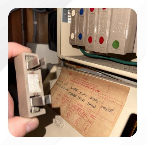
An old fusebox with rewirable fuses and asbestos flash guards is a clear sign of an outdated electrical installation.
